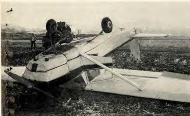
Poor fuel management caused this accident. Pilot and passenger were lucky to escape without critical injuries.
